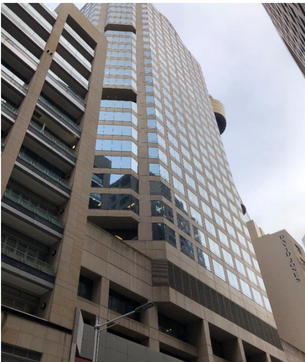
Figure 13 Piccadilly Tower from the south east.
